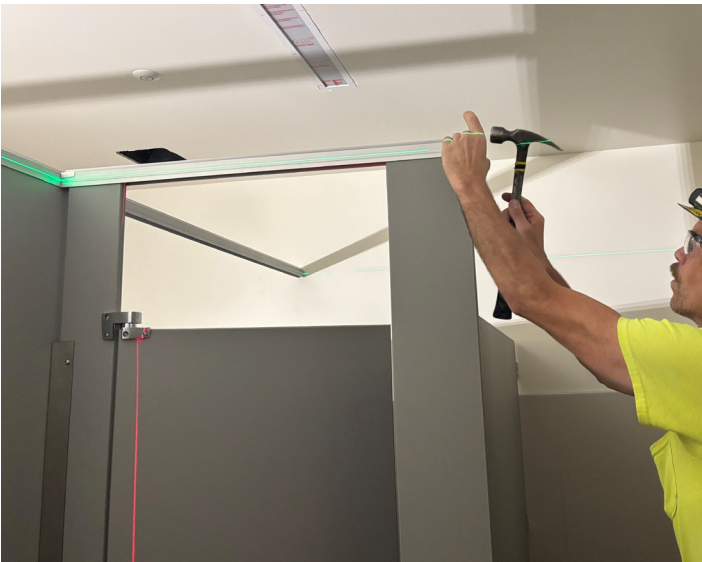
Dupree installing toilet partitions within the Area A lobby bathrooms.
