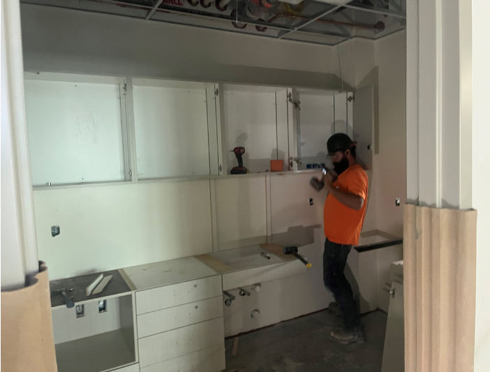
Beck Cabinets installing casework within the Meds room of Residential Inpatient.
